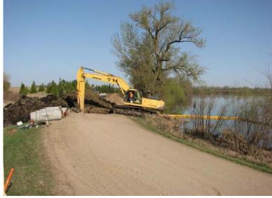
Photo by Matt Olson, DU construction manager <u>Photo Caption</u>: Installing a new water control structure on Jennie Lake in Douglas County
